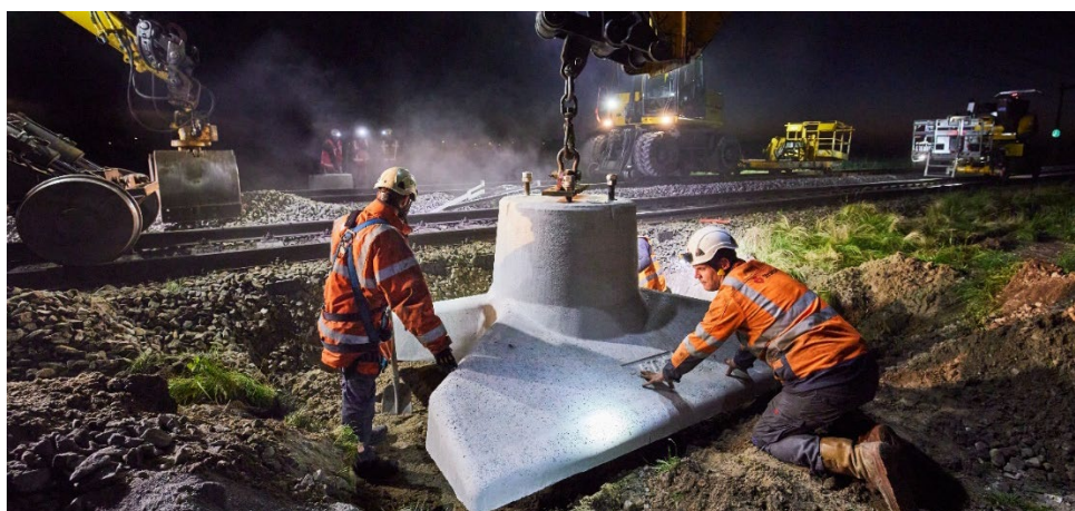
Circular concrete catenary supports
