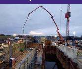
A new pumping station in Zoutkamp to ensure water safety in the area. The renovation of the Hunsingo lock is part of the assignment, as well as the replacement of part of the bank protection.
