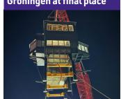
The monumental signal box (90 tonnes) and footbridge (120 tonnes) from 1928 were hoisted into their final place at Groningen Central Station.
