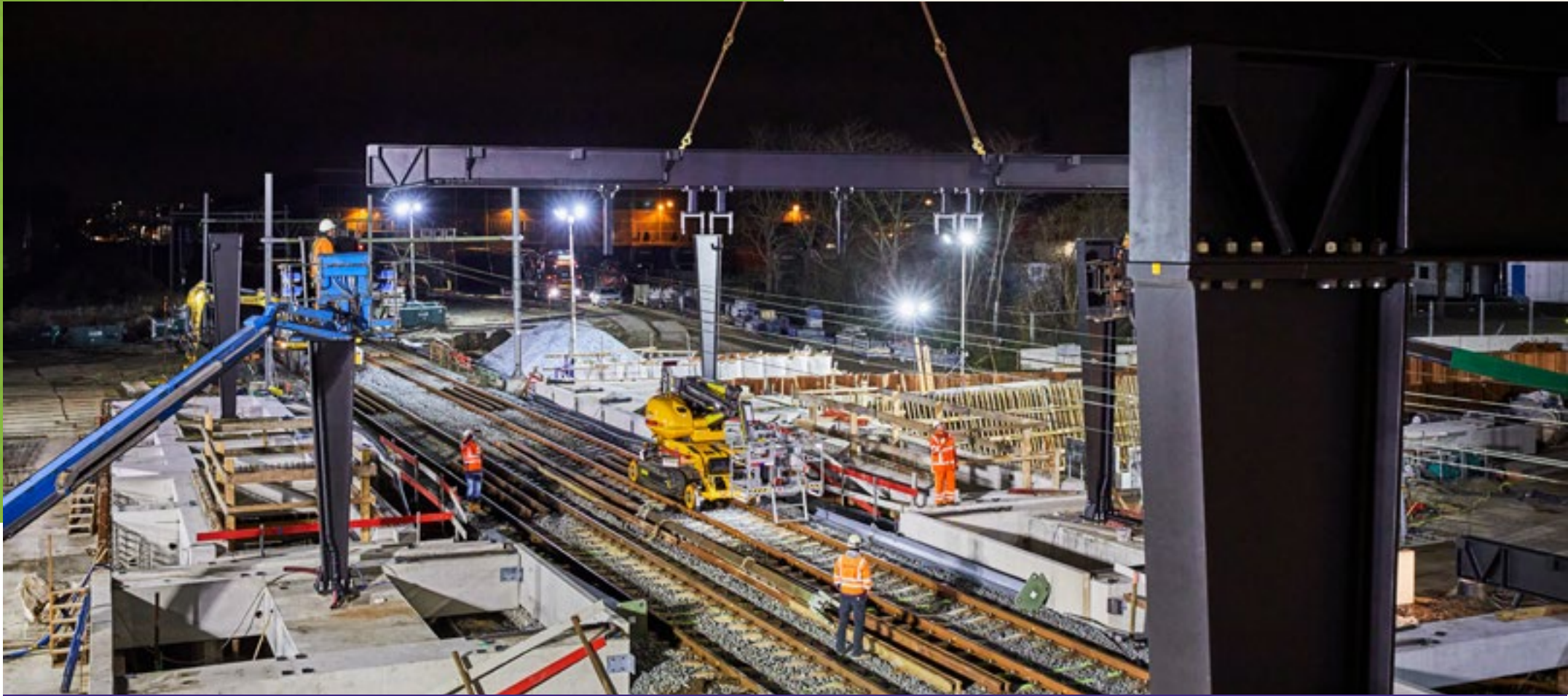
The first poles for the platform roof being installed at Delft Campus.
